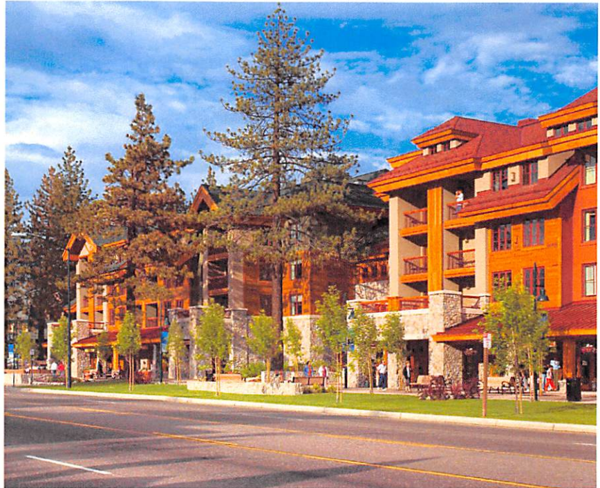
Differentiated materials is one way to visually separate the base floors from the upper floors.
