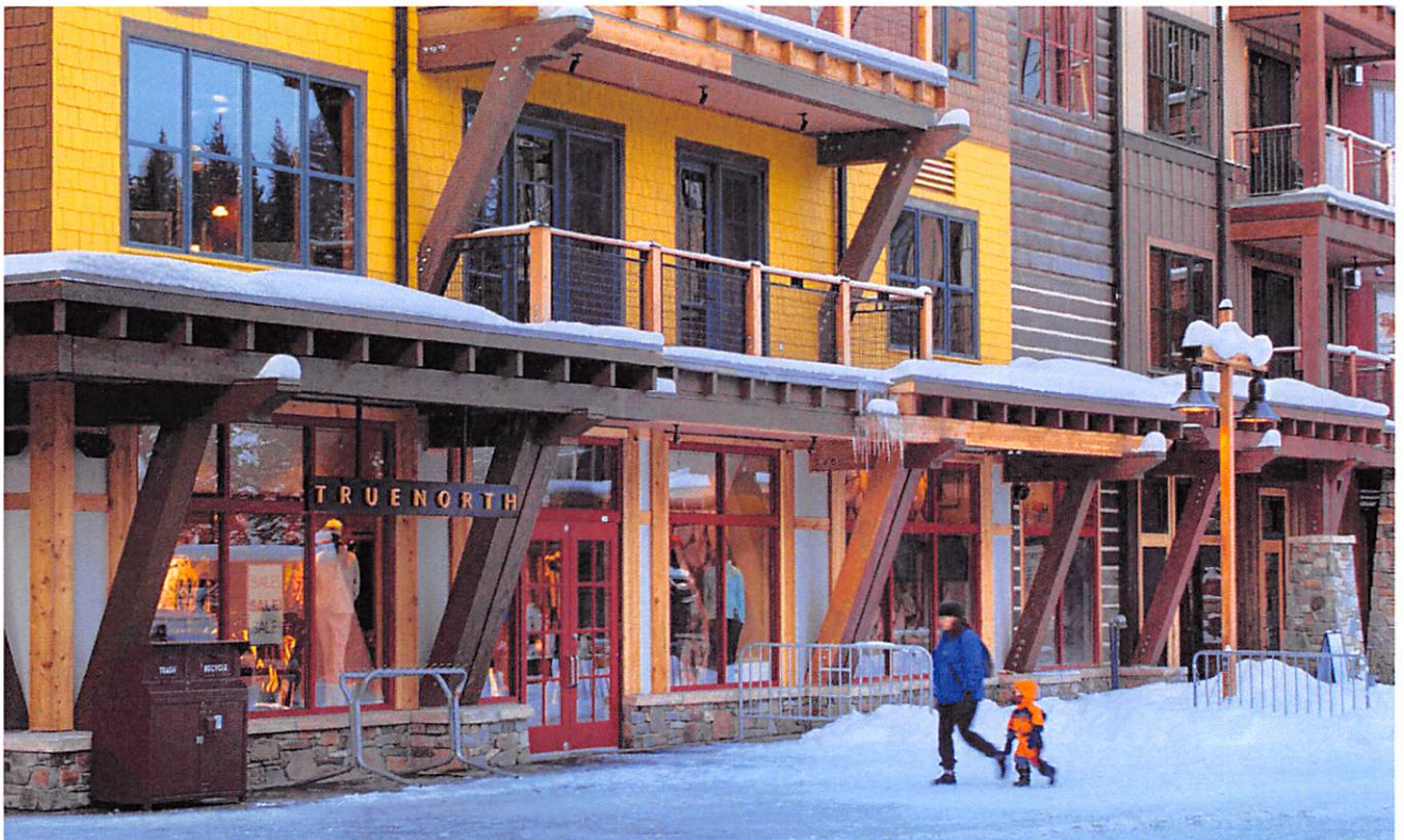
Protruding overhead canopies create interesting architectural façades and provide protection from falling snow.
