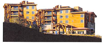
Buildings on natural topography above 15 percent in slope shall be stepped in form.
